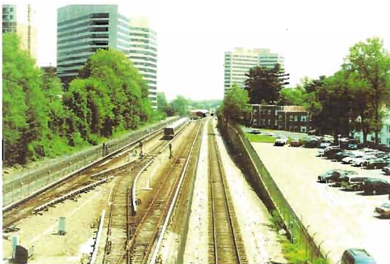
Figure 55: Looking south from Spring Street Bridge
